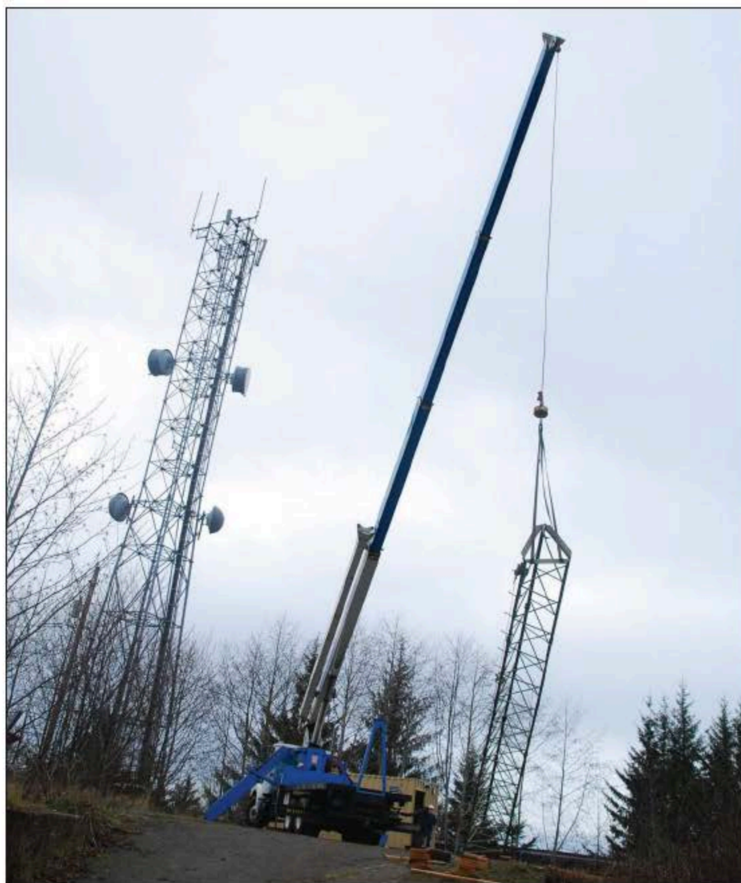
This tower, shown being erected on a mountain peak within the Yurok Reservation, is one of only three new towers necessary for the new TV white-space system being installed.
